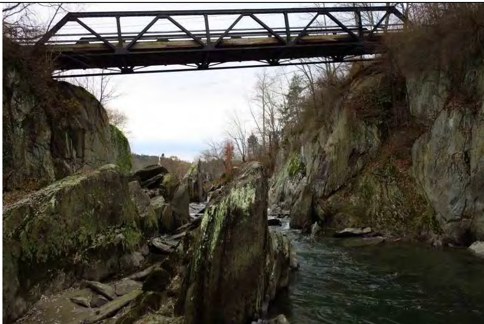
Fletcher Road_B42 outlet of bridge, looking upstream (RS 33765.39)
