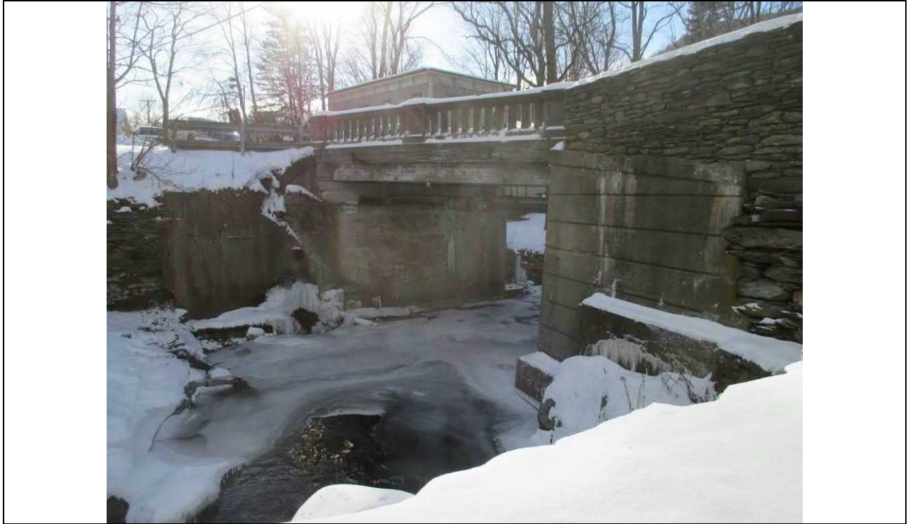
Freeman Brook – Entrance to Main Street bridge in Warren Village (RS 300.40)
