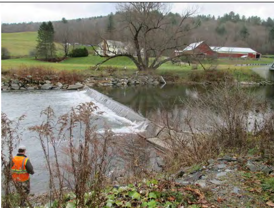
Low dam at USGS Gage downstream of Bridge Road (RS 20933.88)
