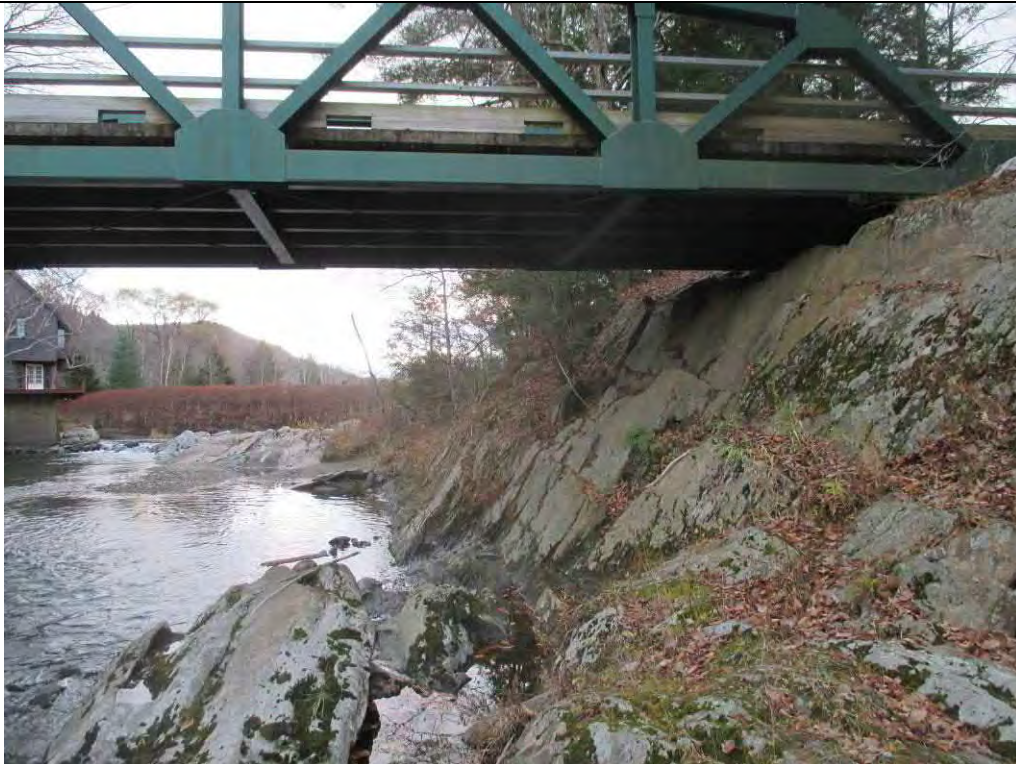
Butternut Hill Road_B22- Looking upstream, left abutment (RS 91019.45)
