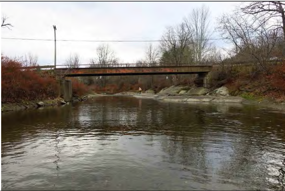
Meadow Road_B24- outlet of bridge (RS 51950.98)
