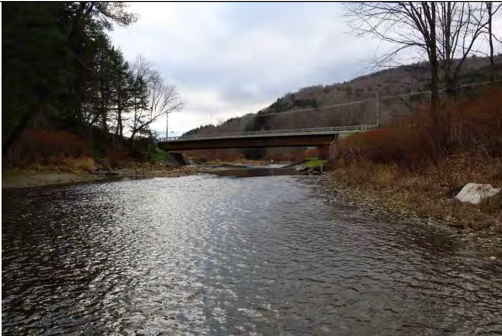
RT100_B177 – Outlet from bridge (RS 81704.02)
