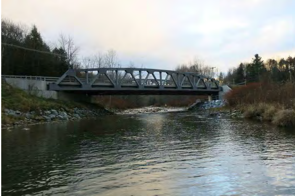
RT100_B173-Outlet to the bridge(Looking upstream) (RS 96377.68)
