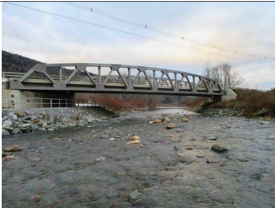
RT100_B173-Entrance to the bridge(Looking downstream) (RS 96377.68)
