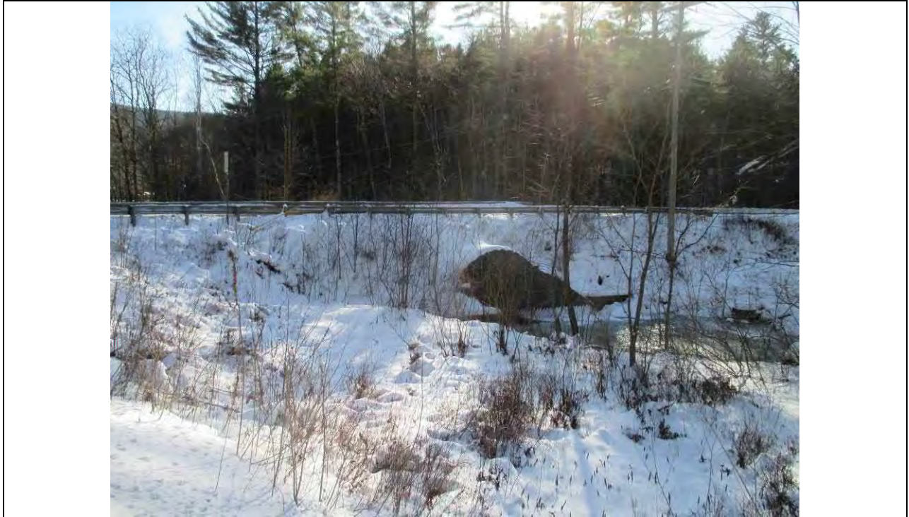
Mill Brook – German Flats Road bridge – entrance to culvert (RS 12181.35)
