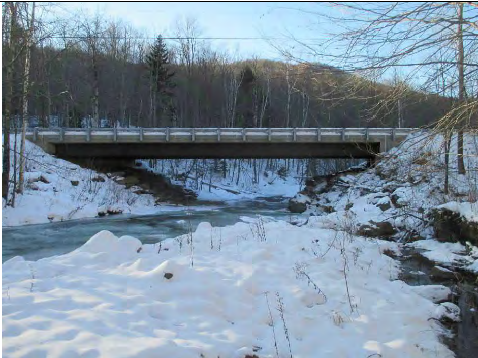
Rt100_B167- Entrance to bridge (RS 122795.8)
