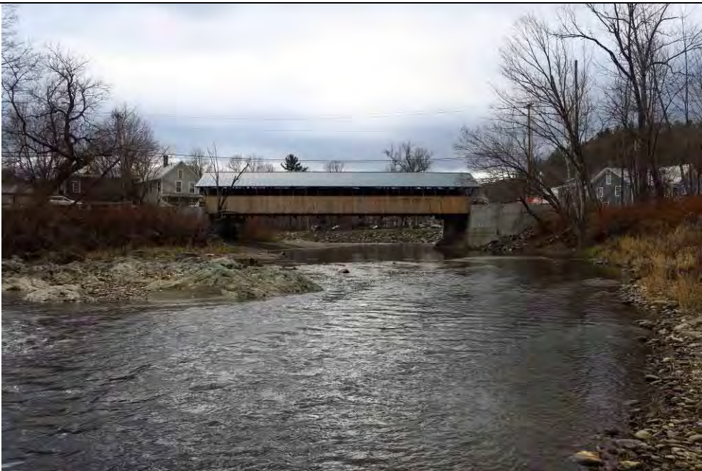
Bridge Street Covered Bridge_CB4- Outlet from Covered Bridge (RS 73267.20)
