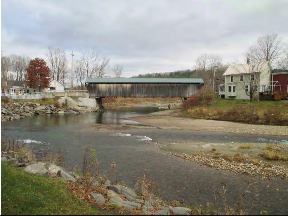
Bridge Street Covered Bridge_CB4- Entrance to Covered Bridge (RS 73267.20)
