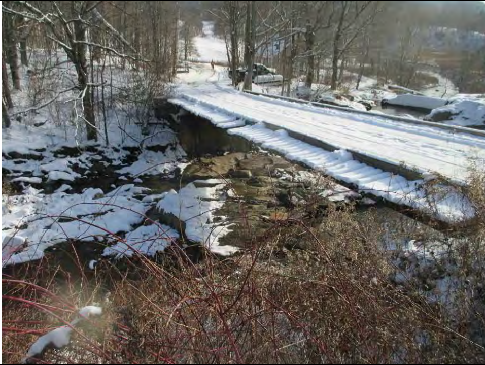
Thatcher Brook – Entrance to Mill Rd bridge (RS 9557.16)
