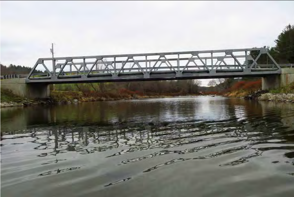
Bridge Road upstream USGS gage, looking upstream. (RS 21081.72)
