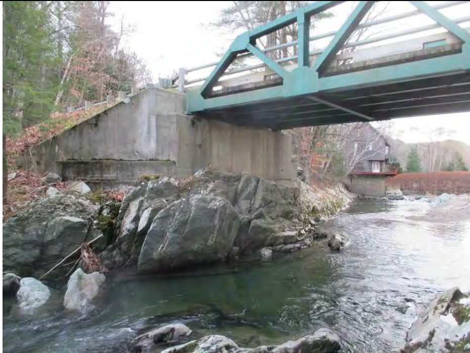
Butternut Hill Road_B22- Looking upstream, right abutment (RS 91019.45)
