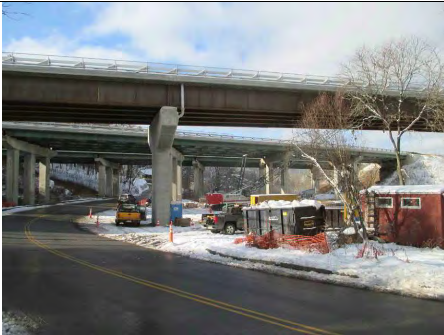
Thatcher Brook – I-89 view looking downstream (Stowe/Waterbury Ramp in the foreground) Ramp has two piers. (RS 4556.90) Ramp (RS 4731.99)
