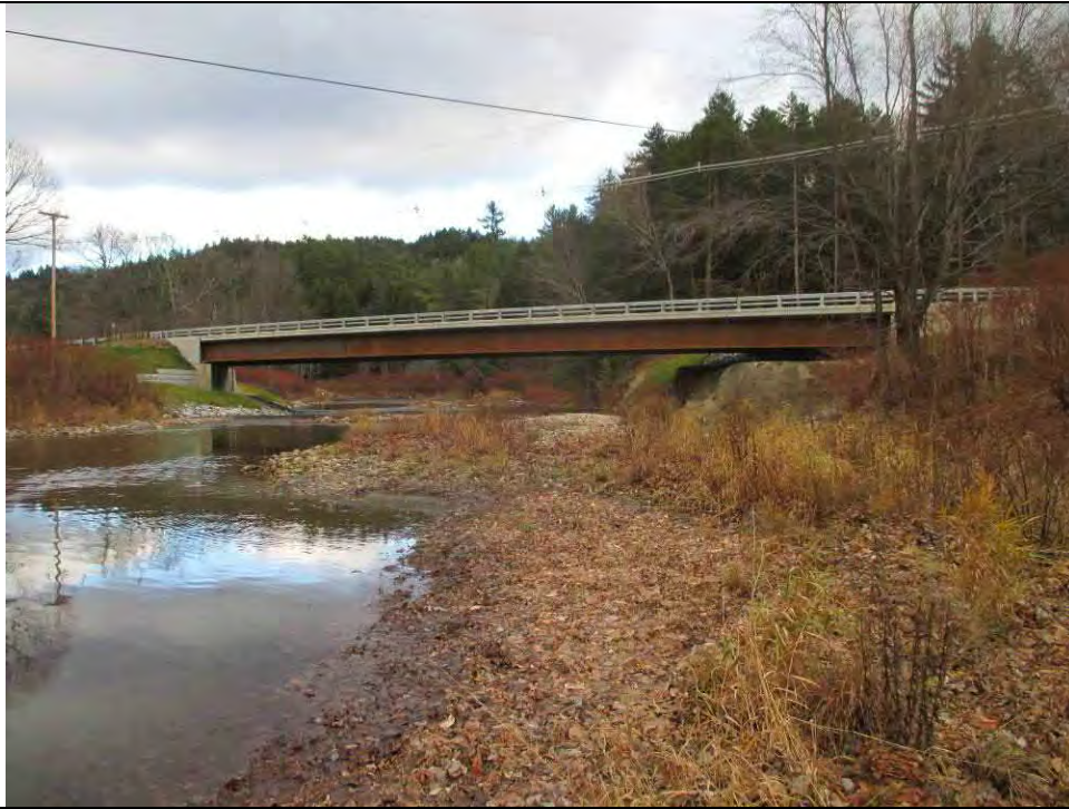
RT100_B177 – Entrance to bridge (RS 81704.02)
