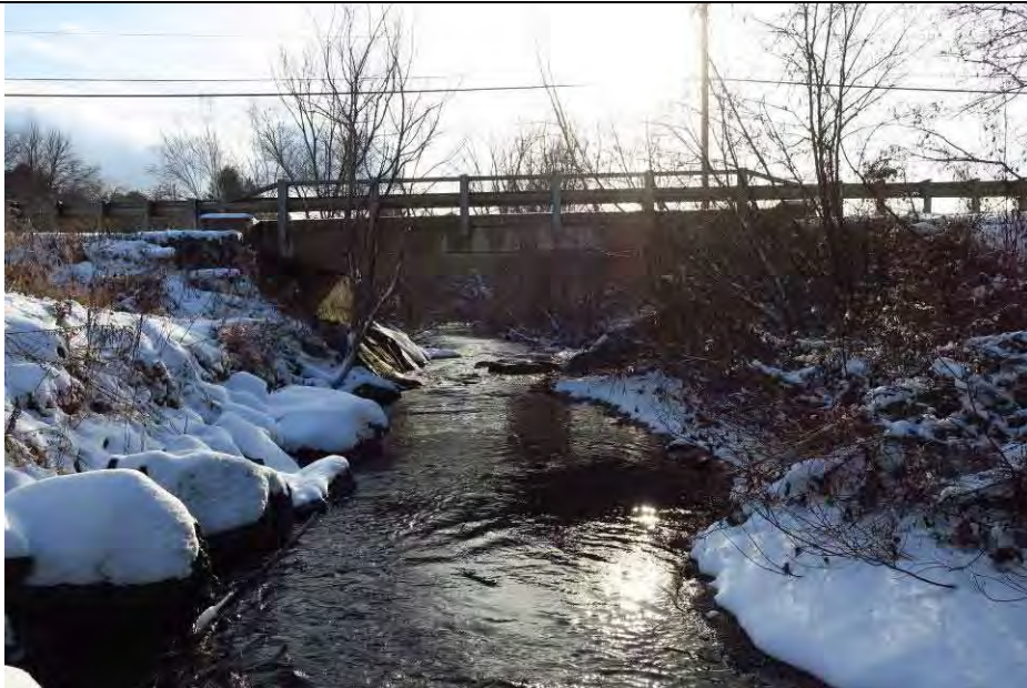
Thatcher Brook – Entrance to Loomis Hill Road bridge (RS 30963.89)
