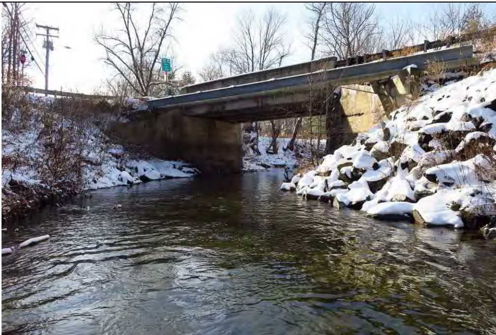
Thatcher Brook – Entrance to Stowe Rd bridge (RS 5970.35)
