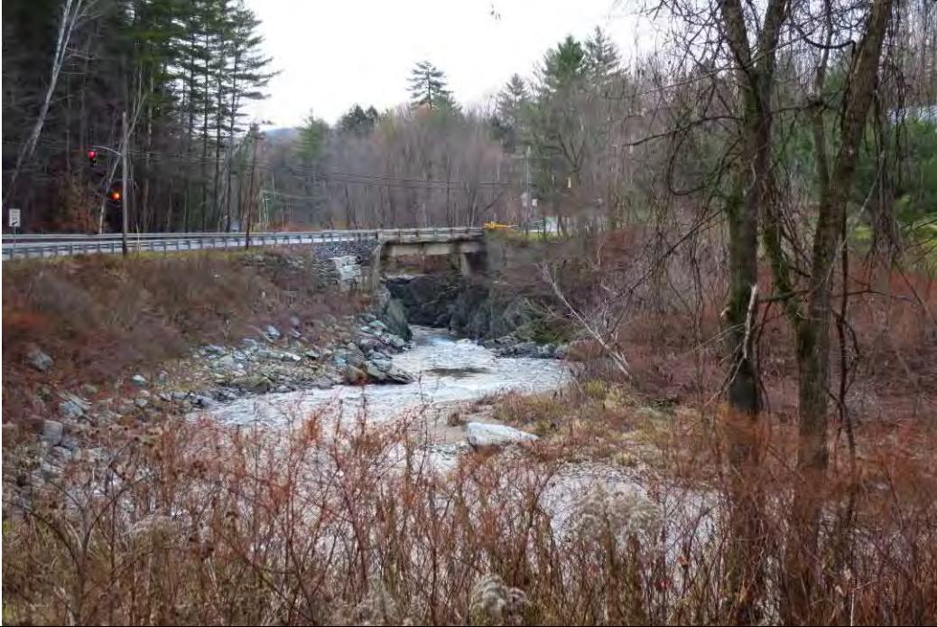
RT110B_B2- Entrance to Bridge, looking downstream (RS 36781.04)
