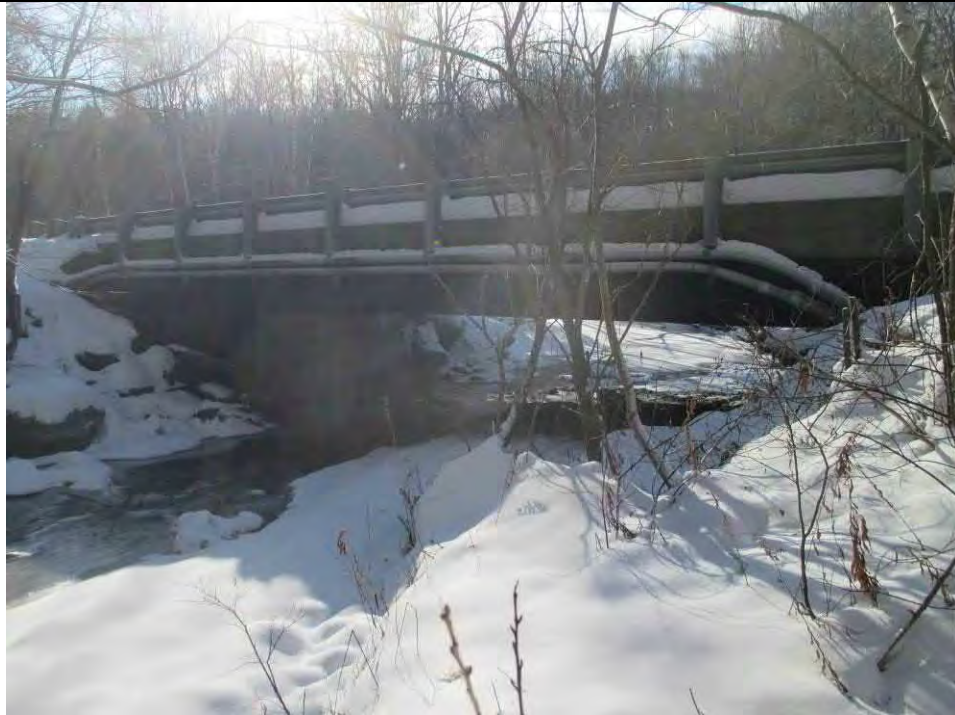
Mill Brook – Mill Brook road (RT17) bridge – entrance to bridge (RS 19247.60)
