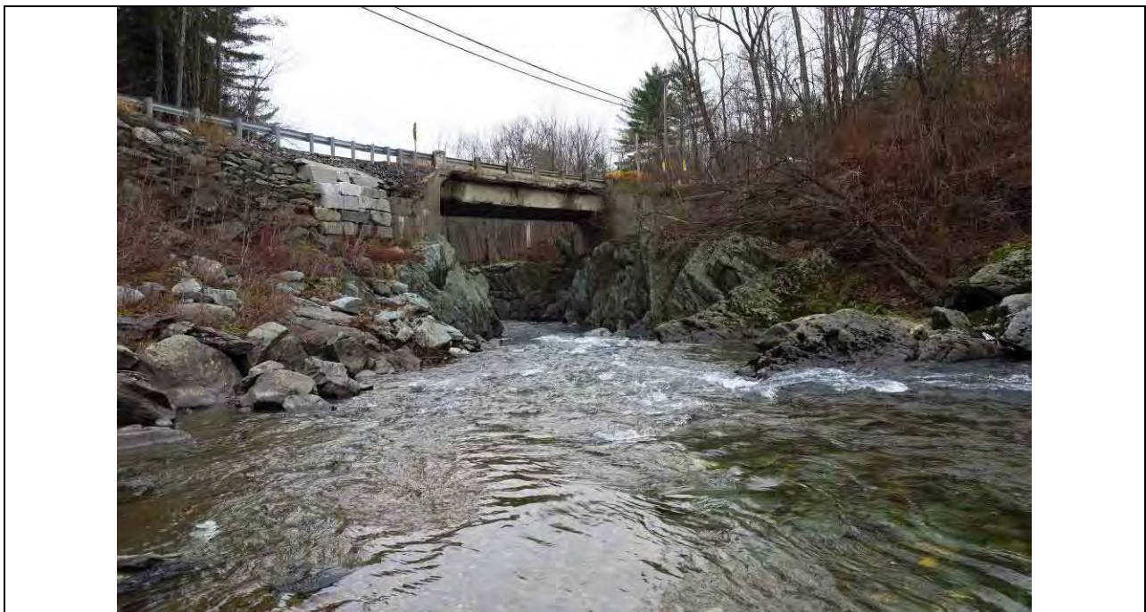
RT110B_B2- Entrance to Bridge, looking downstream (RS 36781.04)
