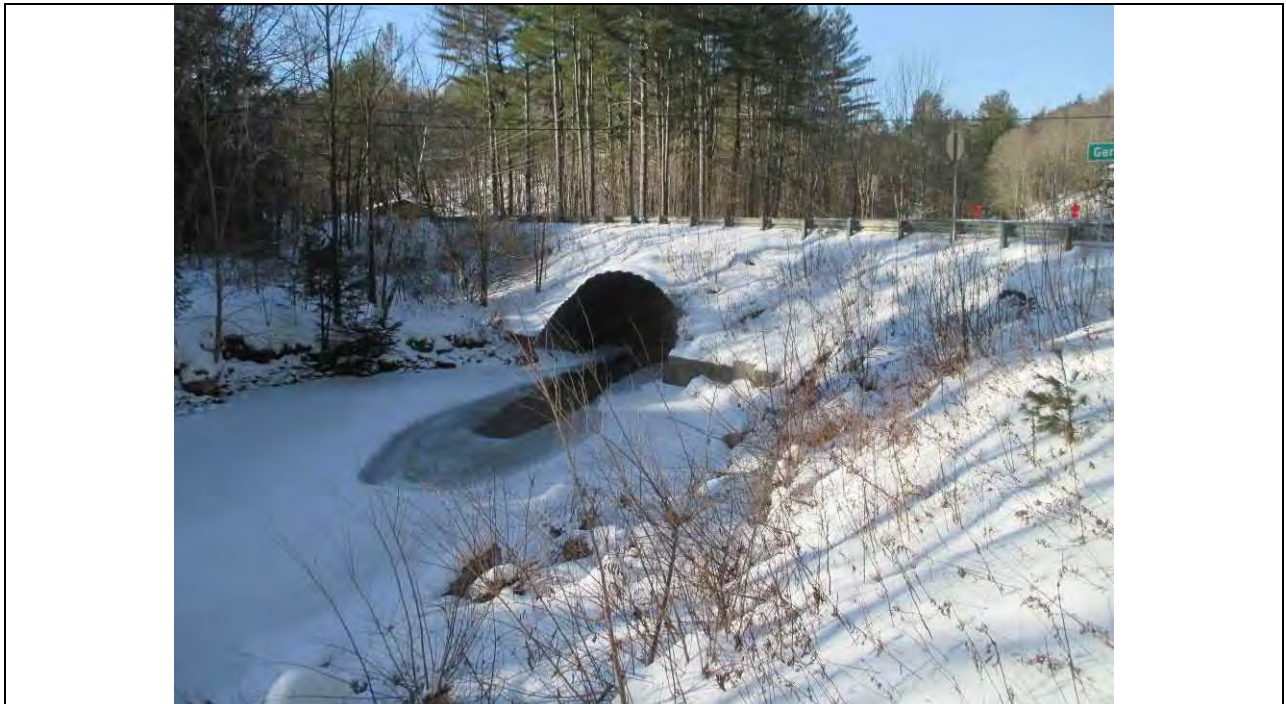
Mill Brook – German Flats Road bridge – outlet of culvert (RS 12181.35)
