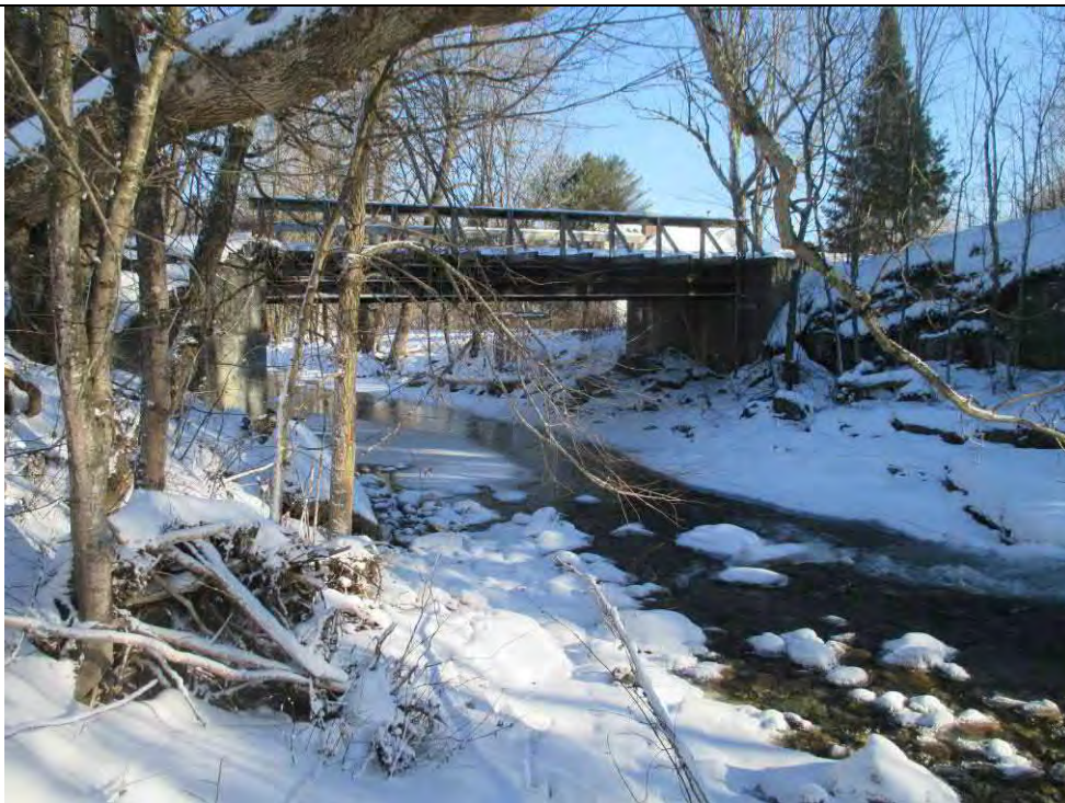
Shepard Brook – Entrance to Private Bridge (RS 1941.68)
