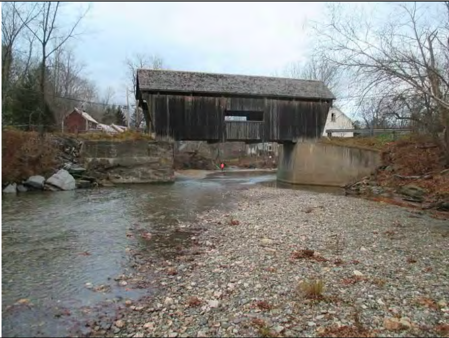
Warren Covered Bridge – Entrance (RS 110006.4)
