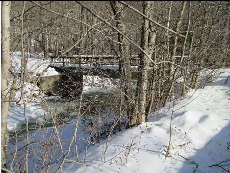
Mill Brook – Private bridge – Entrance to bridge (RS 4504.76)
