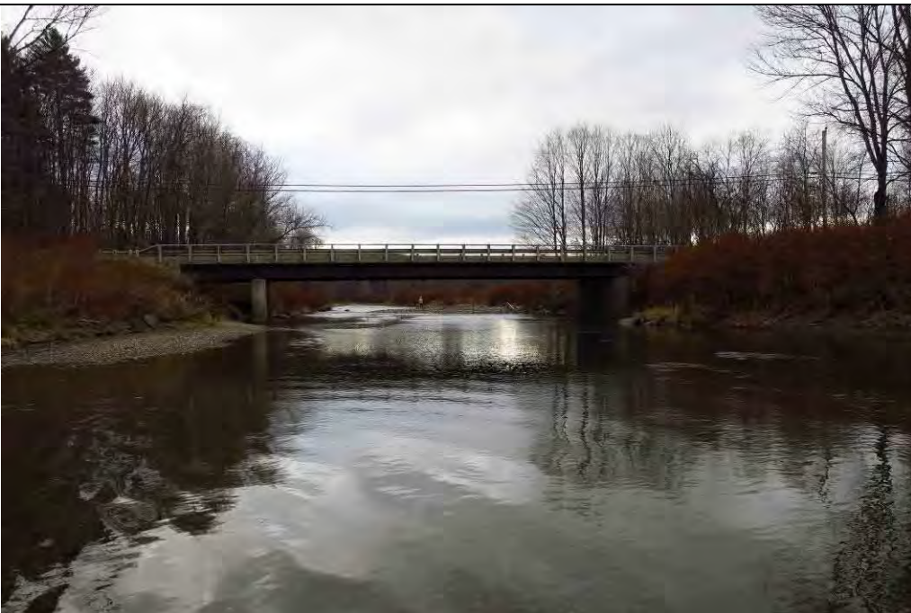
Tremblay Road_B25 – Entrance to bridge (RS 64099.75)
