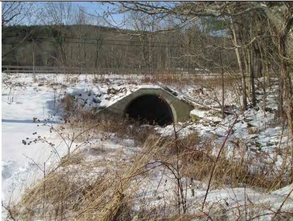
Folsom Brook – Entrance to RT100 culvert (RS 462.75)
