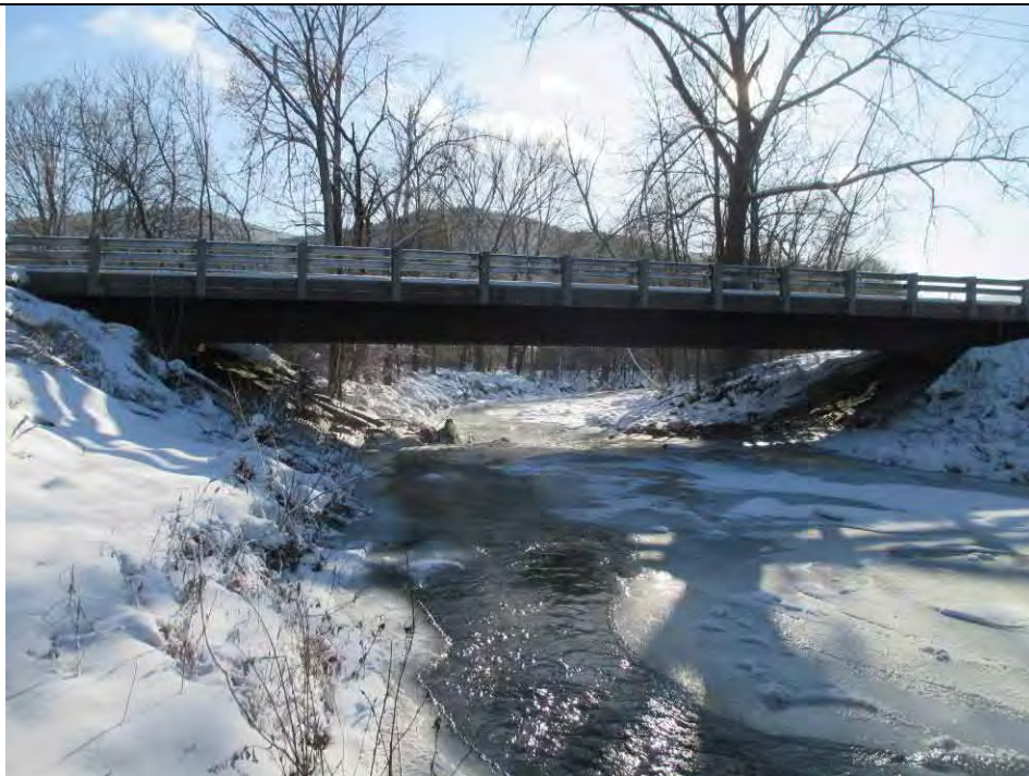
Shepard Brook – RT 100 - Entrance to bridge (RS 939.49)
