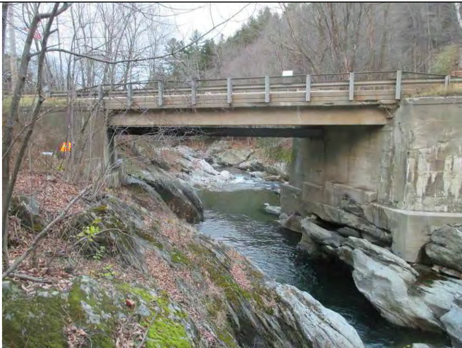
Main Street_B30- Entrance to bridge (RS 107786.8)
