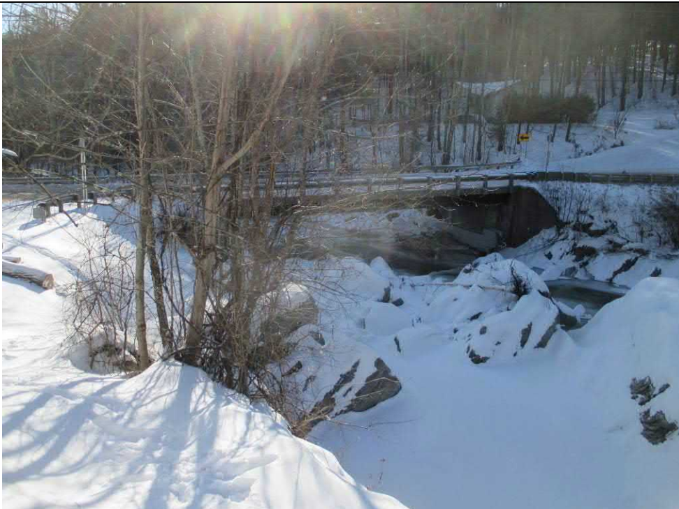
Mill Brook – RT17 – Entrance to bridge (RS 2954.57)
