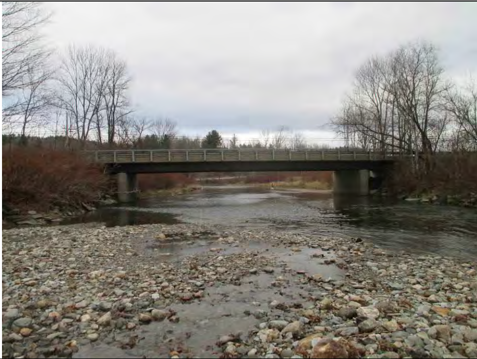
Tremblay Road_B25 – Entrance to bridge (RS 64099.75)
