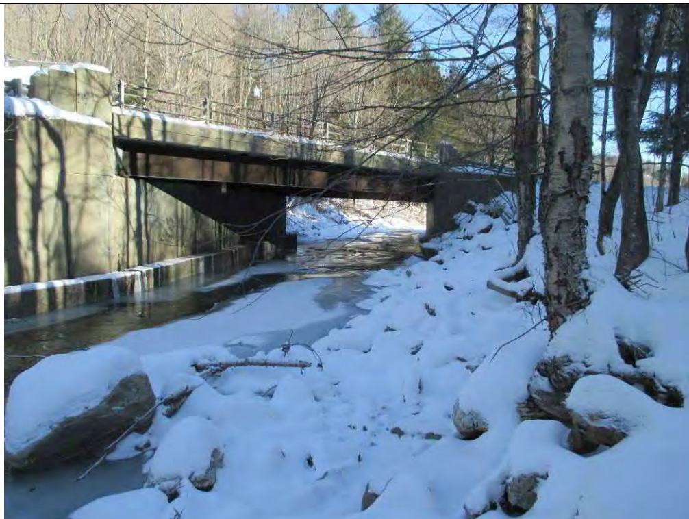
Mill Brook – Mill Brook Road (RT17) bridge No. 01- Entrance to bridge (RS 7688.50)
