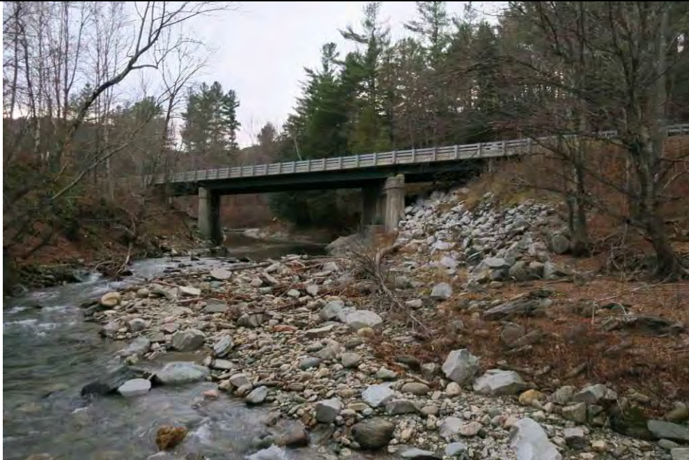
Rt100_B169- Outlet of bridge (RS 112101.0)
