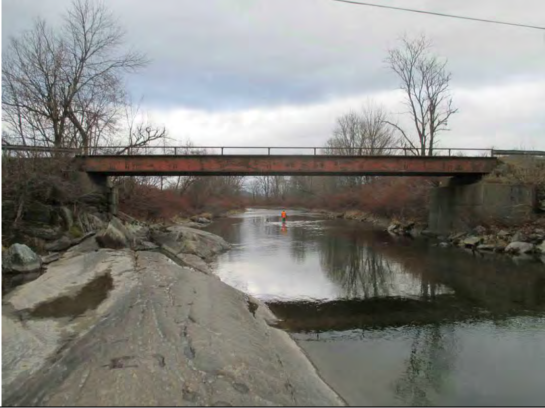
Meadow Road_B24- Entrance to bridge (RS 51950.98)
