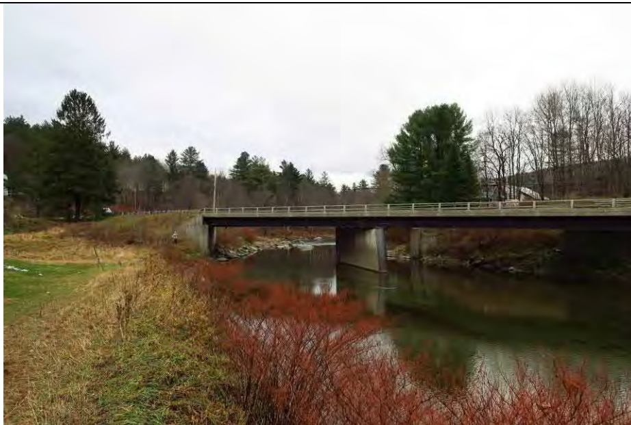
RT110B_B4 – Entrance to bridge, left overbank (RS 31326.51)
