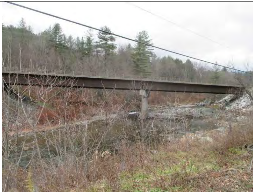
RT110B_B7 – Entrance to bridge (RS 6161.17)
