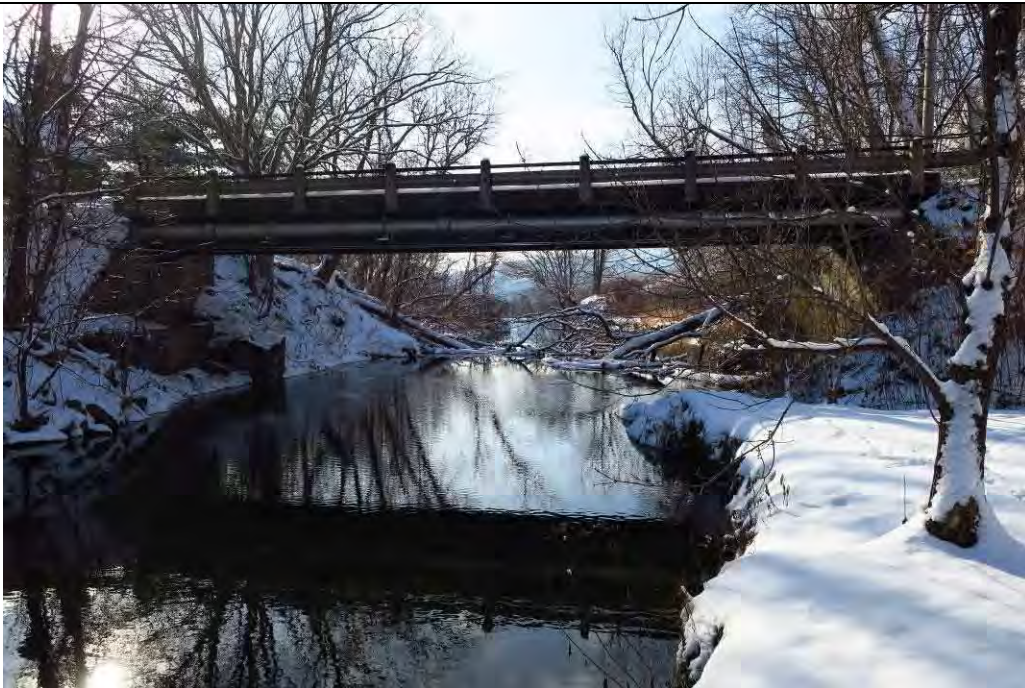
Thatcher Brook – Entrance to Laurel Lane bridge (RS 10001.77)
