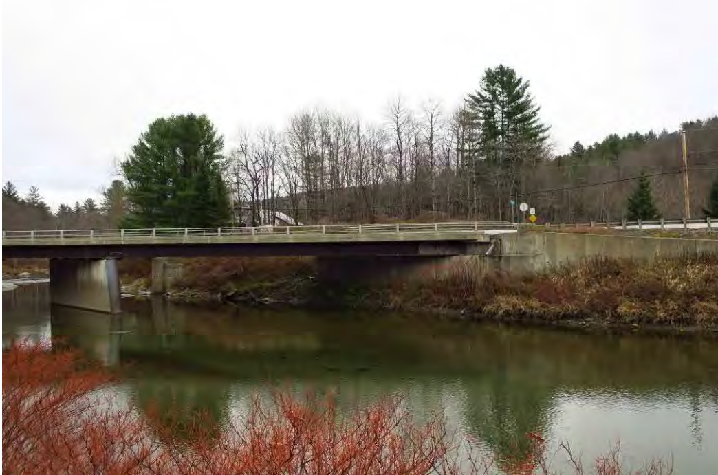
RT110B_B4 – Entrance to bridge, right overbank (RS 31326.51)
