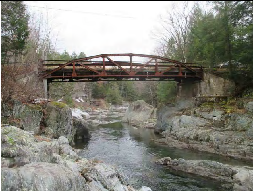
Demas Road – Entrance to bridge (RS 1665.91)
