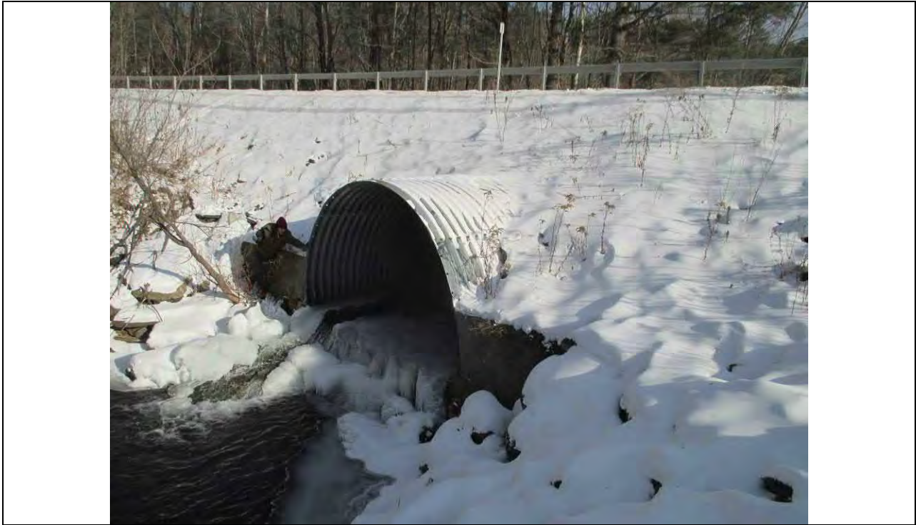
Folsom Brook – Outlet of the RT100 culvert (RS 462.75)
