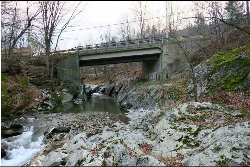
Main Street_B30- outlet from bridge (RS 107786.8)
