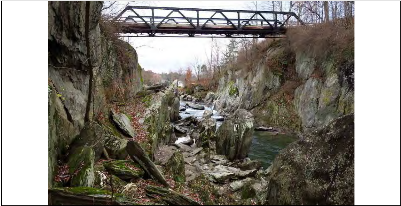
Fletcher Road_B42 outlet of bridge, looking upstream (RS 33765.39)
