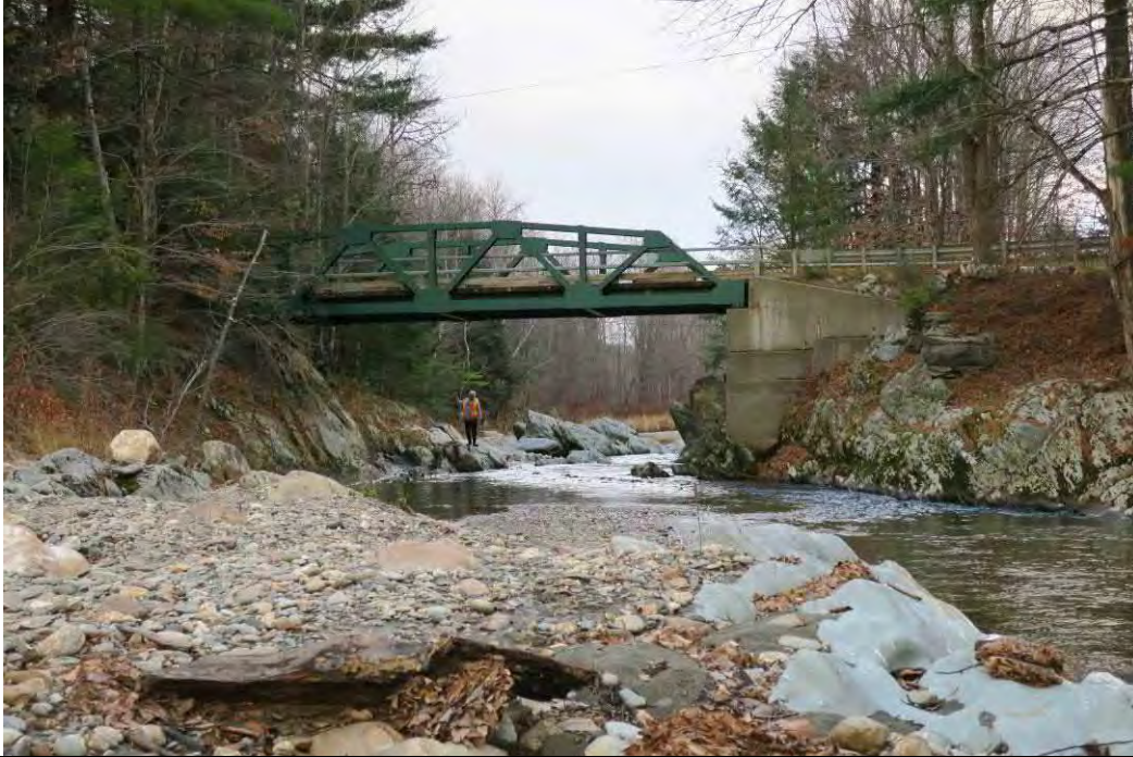
Butternut Hill Road_B22- Entrance to bridge (RS 91019.45)
