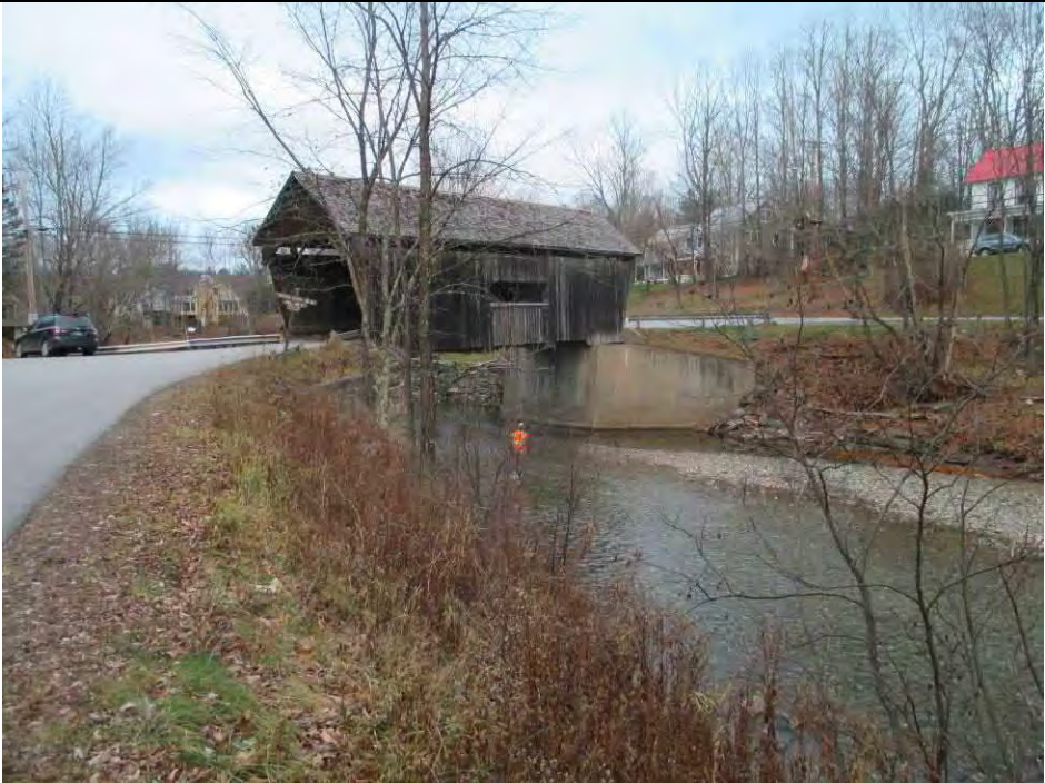
Warren Covered Bridge – Outlet (RS 110006.4)
