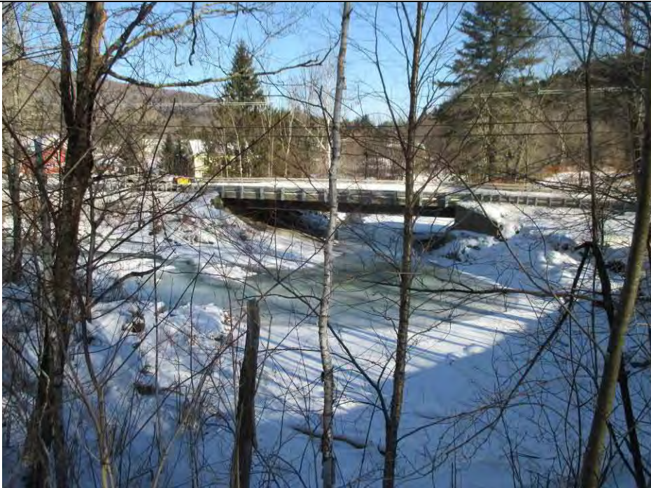
Mill Brook – RT100 – Entrance to bridge (RS 822.25)
