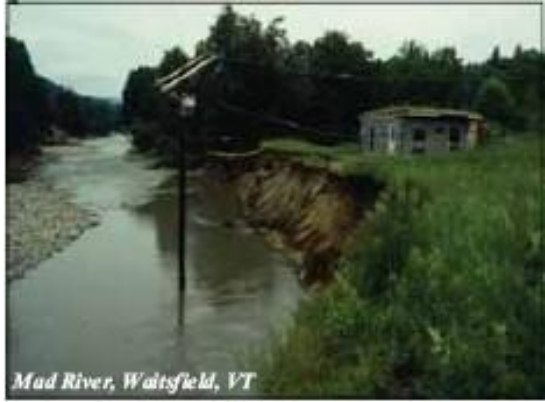
Courtesy of VTDEC River Management Program Fluvial erosion along the Mad River, Waitsfield, Vermont. Image courtesy of VTDEC River Management Program.
