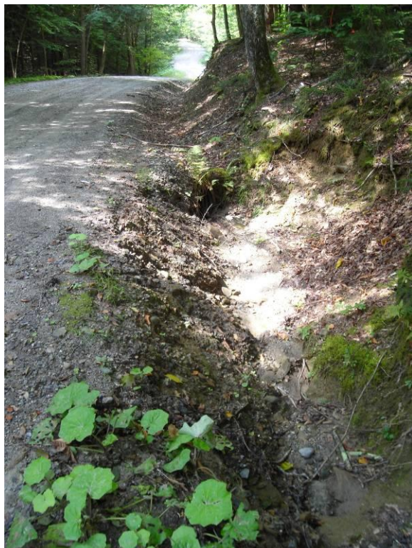
Photos of Site
