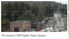
The historic GMP Hydro Power Station
