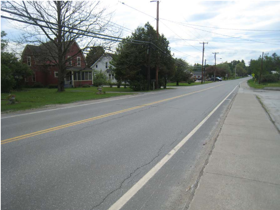
Looking west on Route 2; the narrowing of the paved shoulder from three feet to one foot can be seen just past the driveway entrance on the right side of the road.
