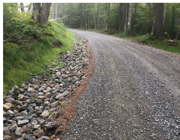
Calais - Apple Hill Road south end one year after BMP installation
