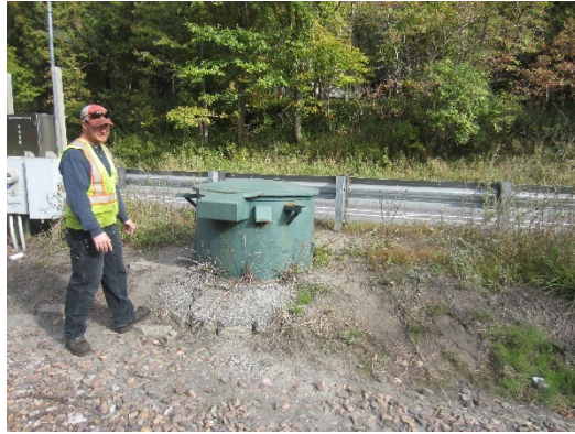
Existing Water Oil/Debris Trap (Approx. MP 6.50)
