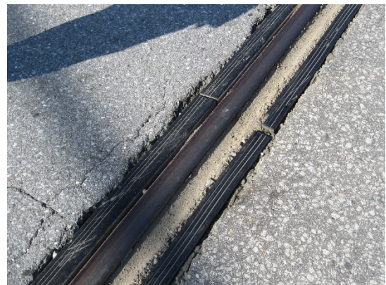
At-Grade Crossing Track with Rubber Rail Seal (Junction Road)
