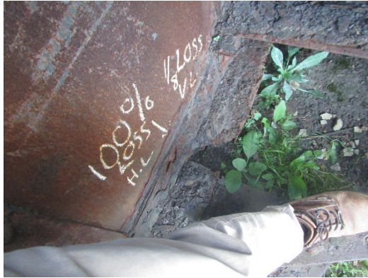
WACR Bridge 306 – 100% Section Loss to End Floor Beam Bottom Flange Horizontal Angle
