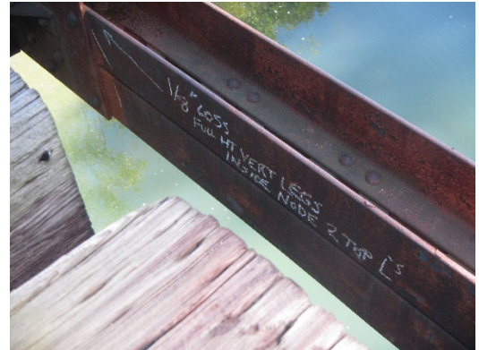
WACR Bridge 307 – Minor Section Loss to Truss Bottom Chord
