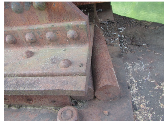
WACR Bridge 303 Expansion Bearing with Dislodged Roller
