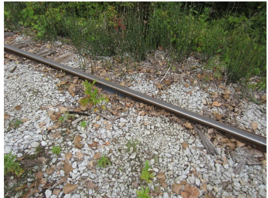
Existing Track Condition – Ballast and Rail
