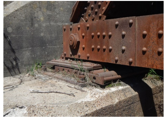
WACR Bridge 306 – Expansion Bearing with Partially Ejected Roller Nest
