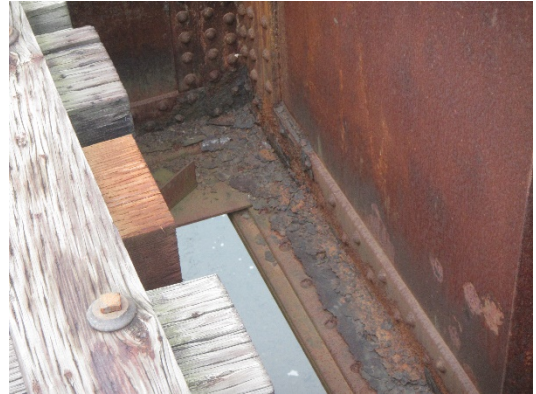
NECR Bridge of the Dog River – Corrosion with Section Loss to Floor Beam to Girder Connection and Girder Bottom Flange
