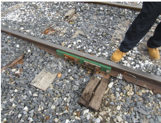
Existing Insulated Joint for Gin Lane Flashers
