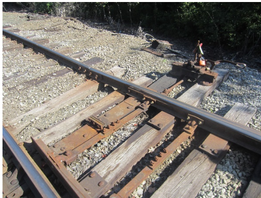
Existing Manual Switch at No. 8 Turnout
