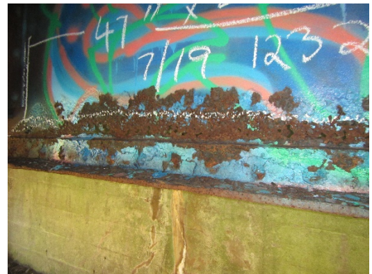
WACR Bridge 305 – Typical Section Loss to Stringer at Bottom of Web
