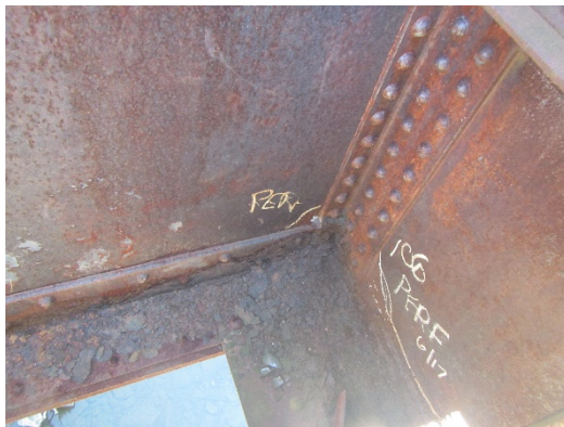
WACR Bridge 305 – Girder and Floor Beam Perforations at Floor Beam to Girder Connection
