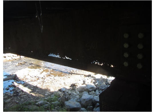
WACR Bridge 304 – Typical Section Loss to Stringer at Bottom of Web
