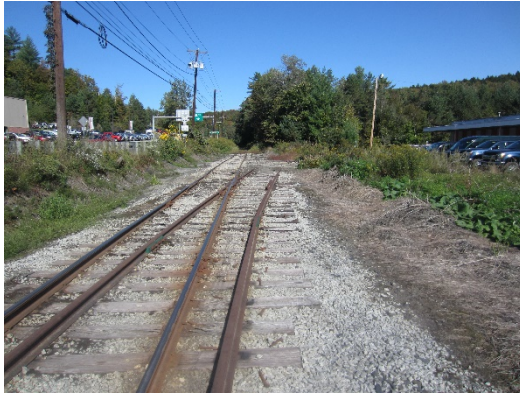
Existing No. 8 Turnout before Vacant Lot Crossing (Facing North)
