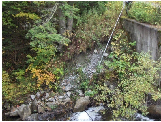
Figure 7.30. Mass failure at Apple Hill Road crossing in T3.08SI.04-A
