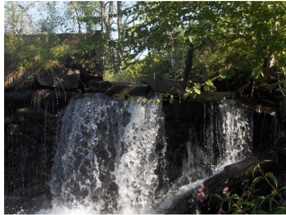
Figure 7.10. Old rock dam in T3.09 causing grade control and channel constriction
