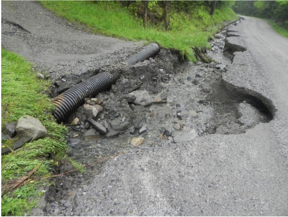
Figure 2: Beaver Meadow Rd damage from May 2011 flood. Source: Town of Marshfield
