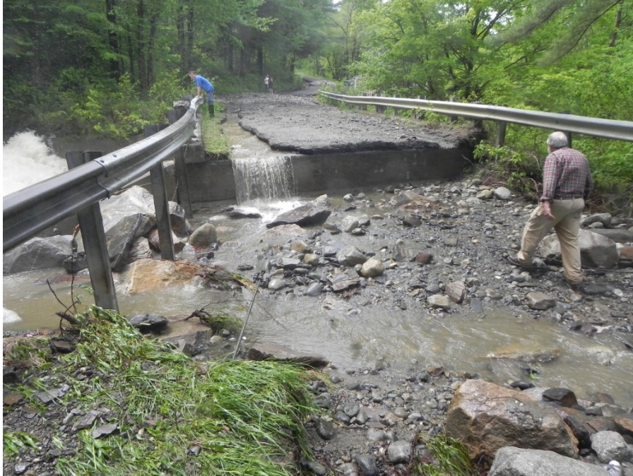
2 Figure 6: Lower Depot Rd damage from May 2011 flood. Source: Town of Marshfield
