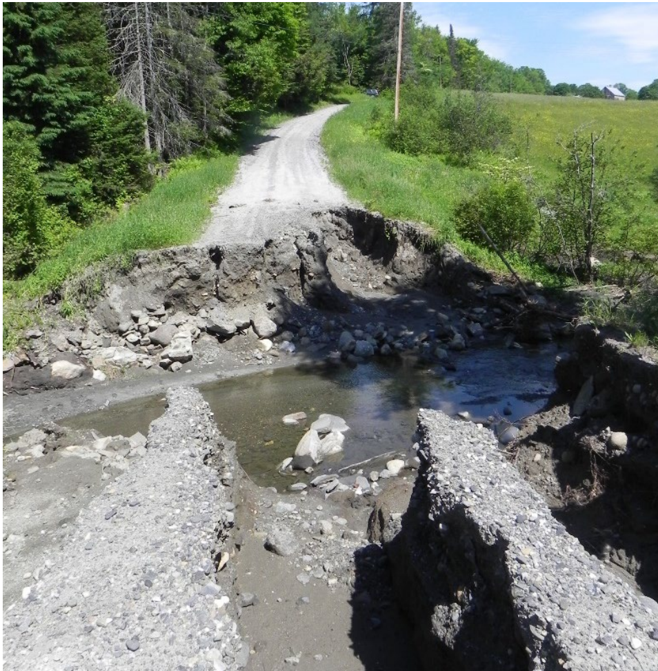
4 5 Figure 9: Jake Martin Rd damage from May 2011 flood. Source: Town of Marshfield
