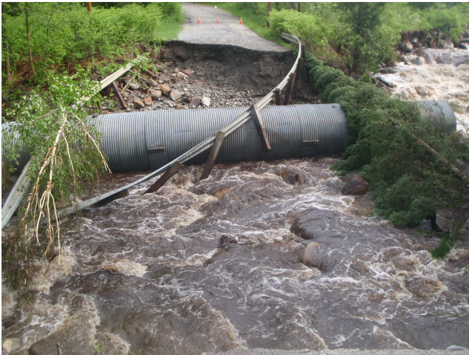
5 Figure 5: Laird Pond Rd damage from May 2011 Flood. Source: Town of Marshfield
