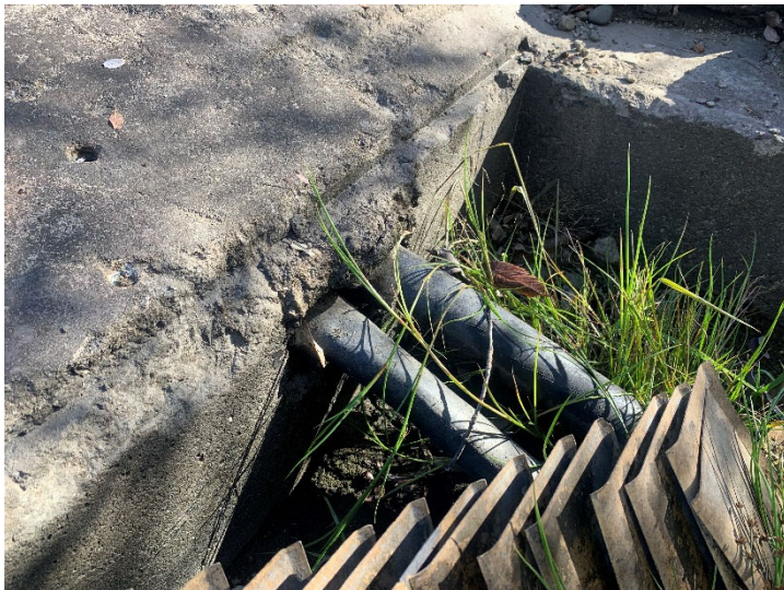
Photo 7: PVC conduit set in concrete at the subject property.
