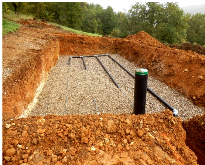
A sand filter under construction.
