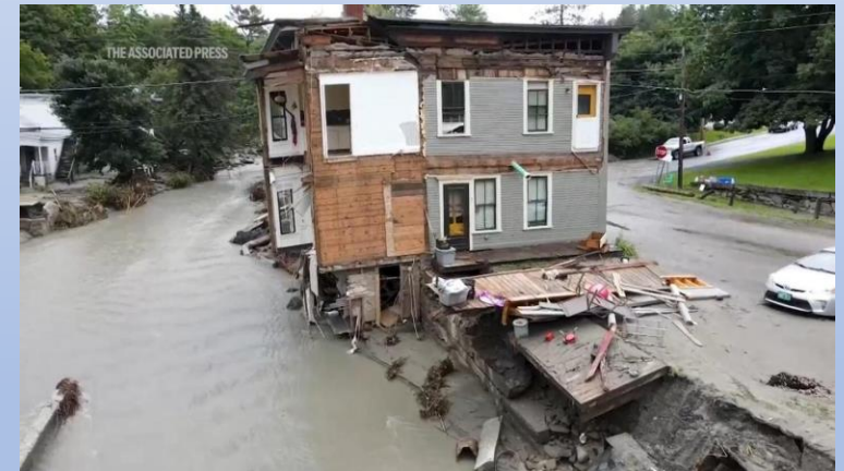
River Corridor Erosion – Plainfield, 2024
