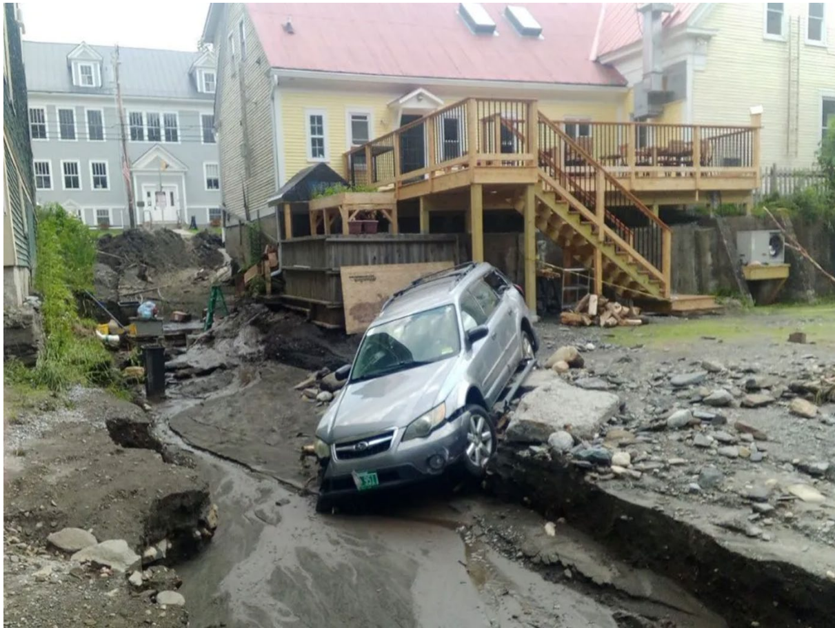
July 2023 Flood Damage
