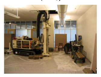
Our probes are track mounted and capable of accessing low clearance and indoor projects.
