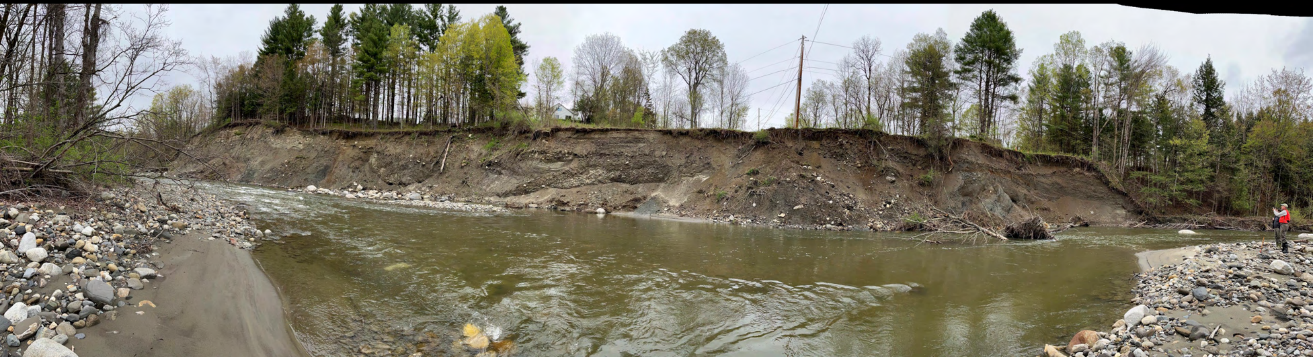
Figure 8: Panoramic photo taken by Jesse Armfield on 5/8/2025. This photo shows the entire failing bank as well as the health center, house, utility pole, and the location of the road on top of the bank to the right of the pole. Note that the image is distorted because it was captured as a panoramic photo.
