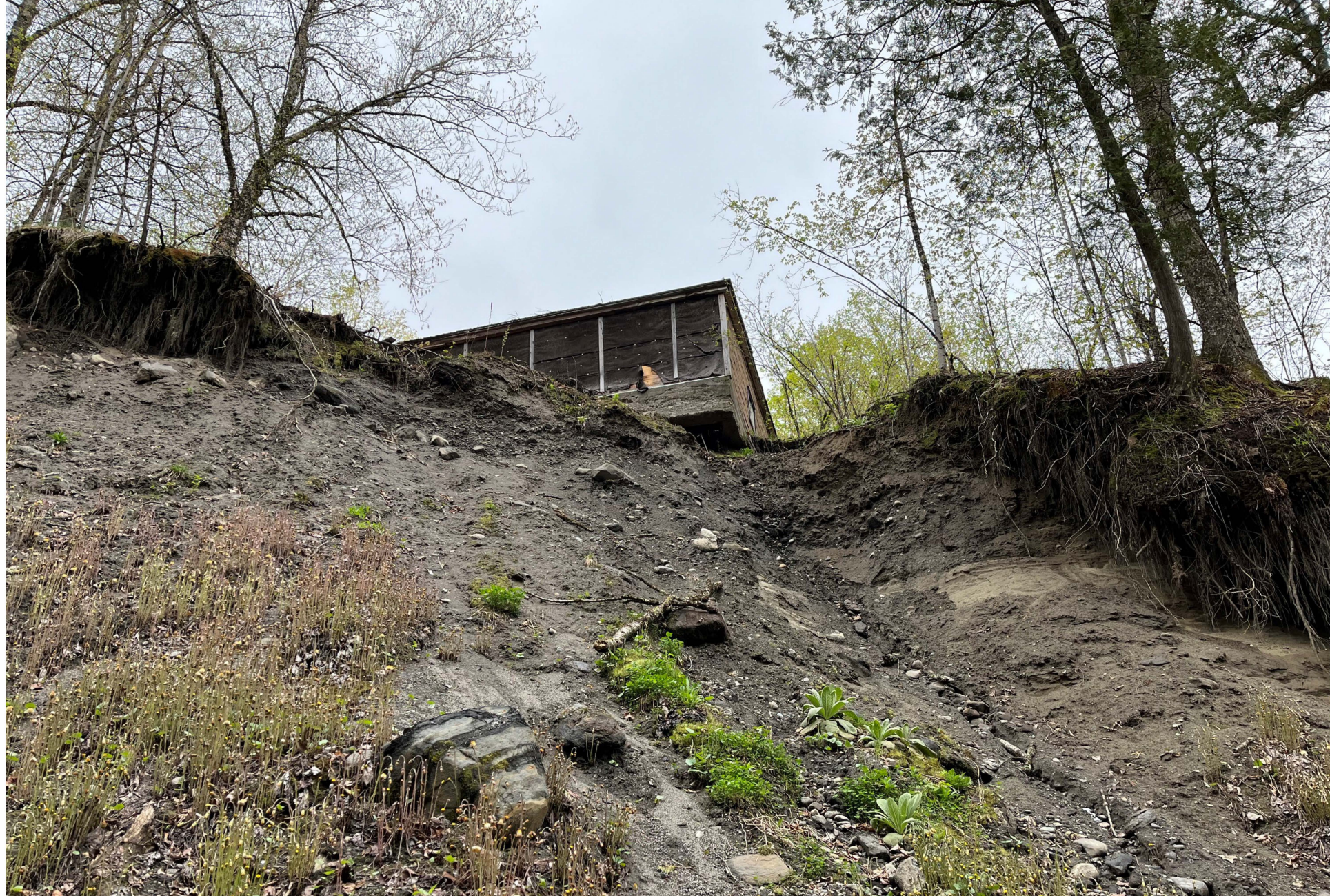
Figure 4: Photo of garage on 5/8/2025. This photo shows the footing of the garage unsupported by soil. This photo also shows the small channel/rill forming below this structure.
