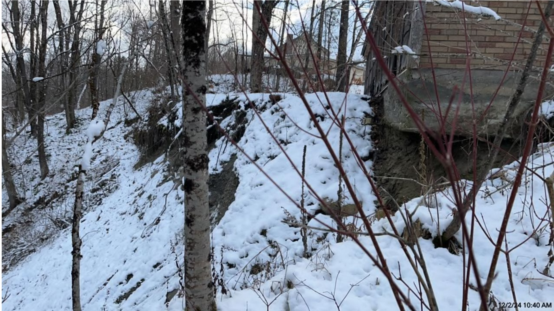
Figure 3: Photo taken on 12/2/2024 showing the garage and slope below. Note that the footing of the garage is exposed but compare this to the exposure in Figure 4.
