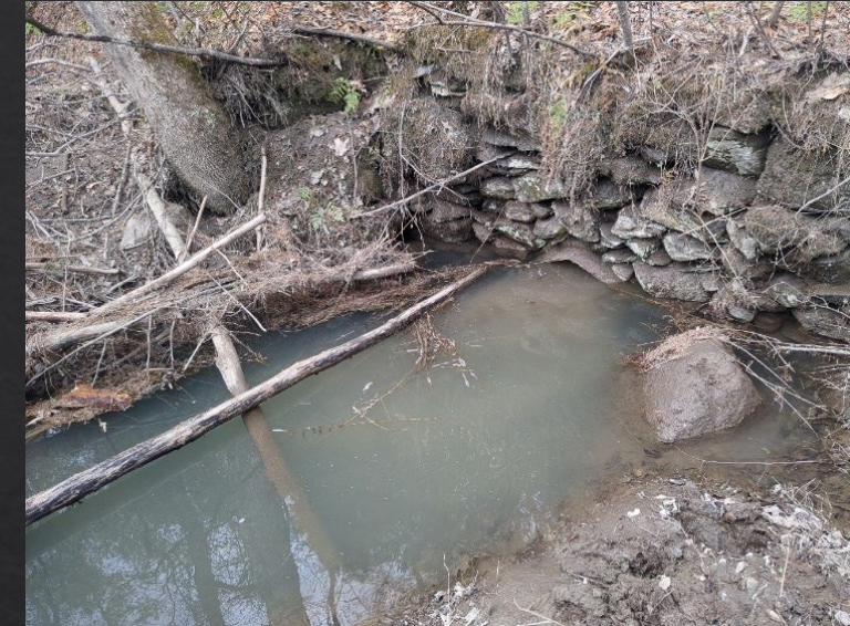
outlet of old road culvert
