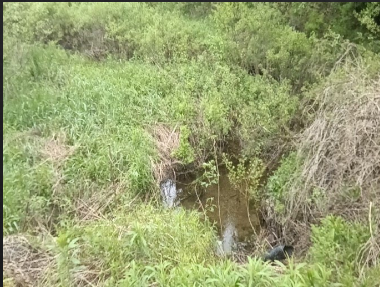
upstream of culvert
