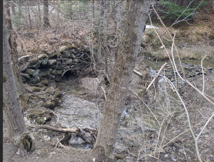
inlet of old road culvert
