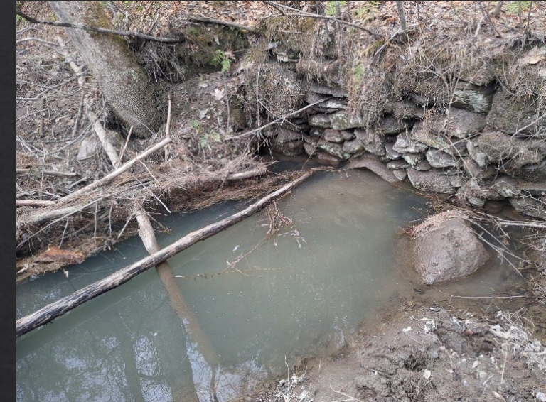
outlet of old road culvert
