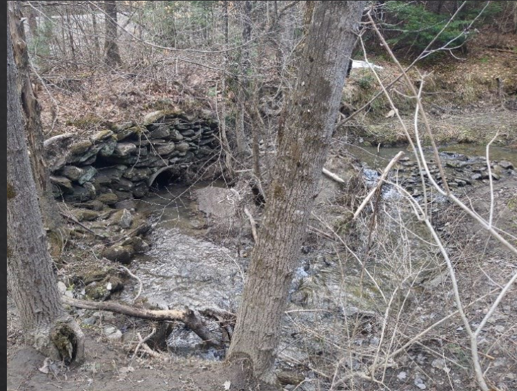
inlet of old road culvert
