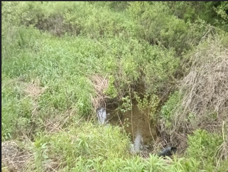
upstream of culvert
